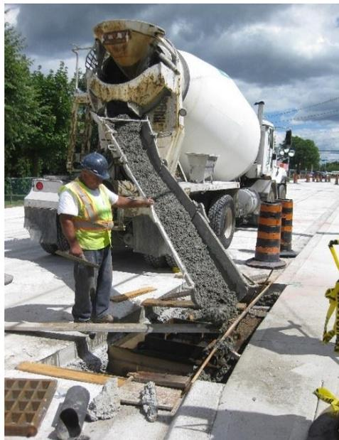
**Figure 4-22 Concrete Poured in box-outs**
