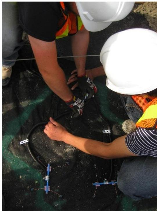
**Figure 4-19 Installation of vibrating wire strain gauges (Section 1)**
