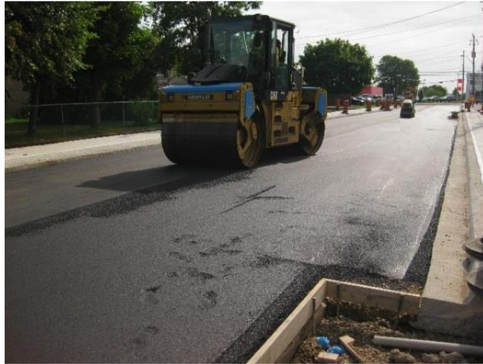
**Figure 4-17 Placement of HMA separation layer**
