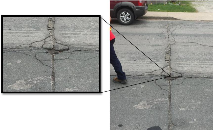
**Figure 3-5 Typical deterioration on transverse saw-cut joints (Pickel, et al., 2016)**
