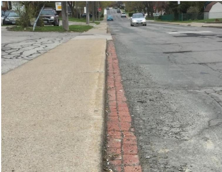
**Figure 3-4 Brick gutter along Jameston Ave. (Pickel, et al., 2016)**
