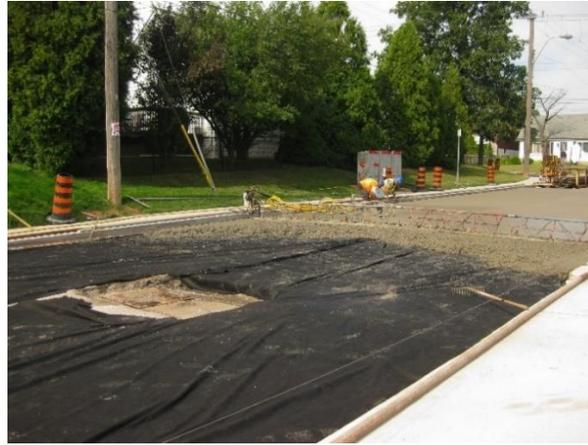
**Figure 4-14 Geotextile cutout for manholes and catchbasins**
