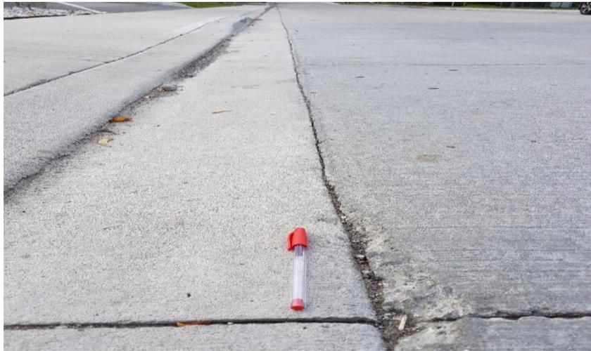
**Figure 5-31 Moderate longitudinal joint spalling – Section 3 – 1Y after construction**
