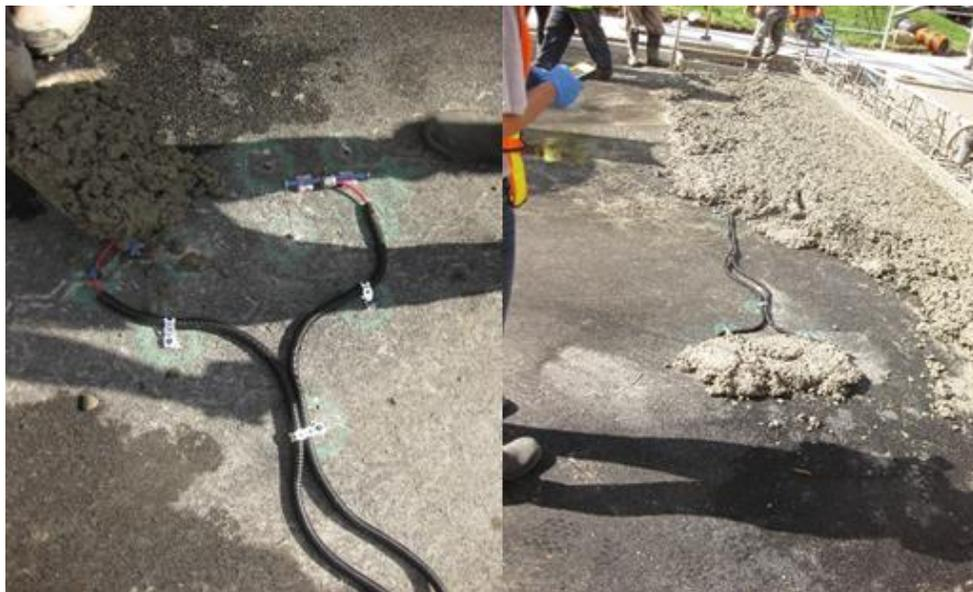
**Figure 4-8 Typical sensors being covered using fresh concrete and cable running across the street**
