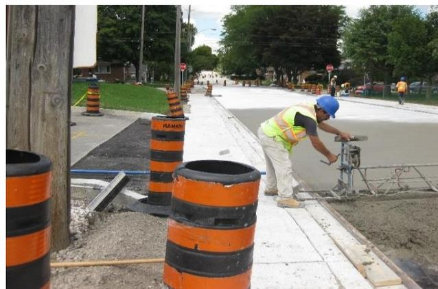
**Figure 4-21 Use of high early strength concrete on Section 3**
