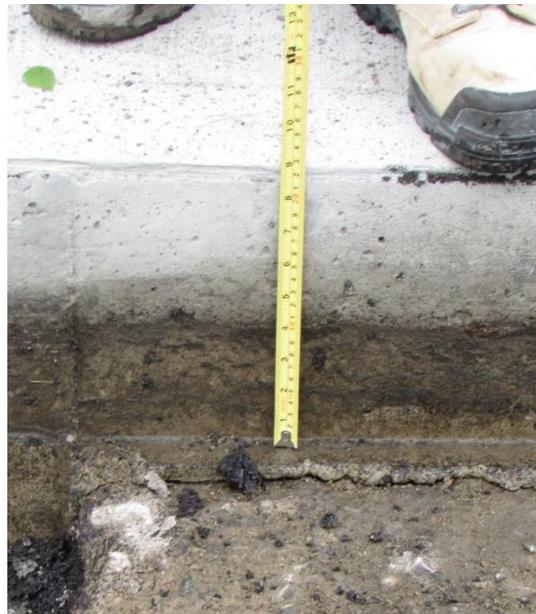
**Figure 4-2 Height from the bottom of existing concrete to top of curb (Section 1) (Pickel, et al., 2016)**
