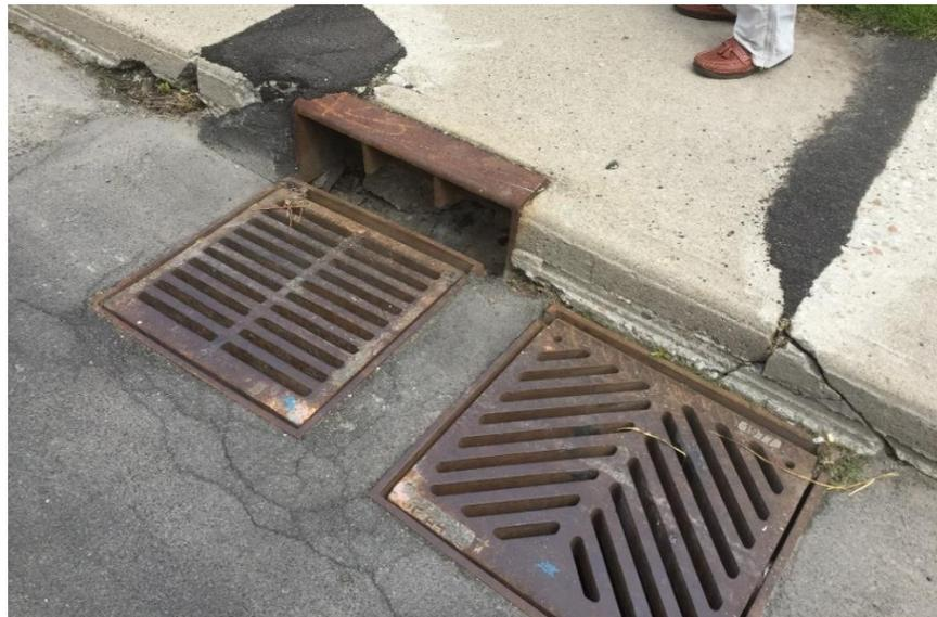
**Figure 3-7 Settled catch basins in Section 2 (Pickel, et al., 2016)**
