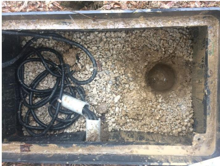
**Figure 4-10 Trench hole and gravel to allow drainage of water – Section 1**
