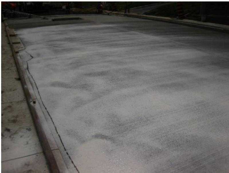
**Figure 4-16 Uneven placement of curing compound**
