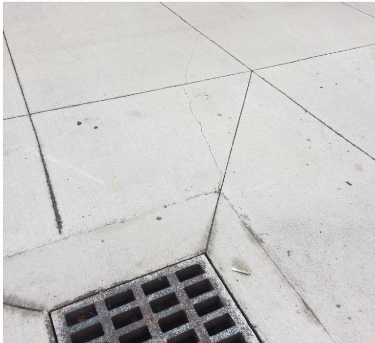
**Figure 4-29 Transverse crack in Section 1 close to catchbasin**
