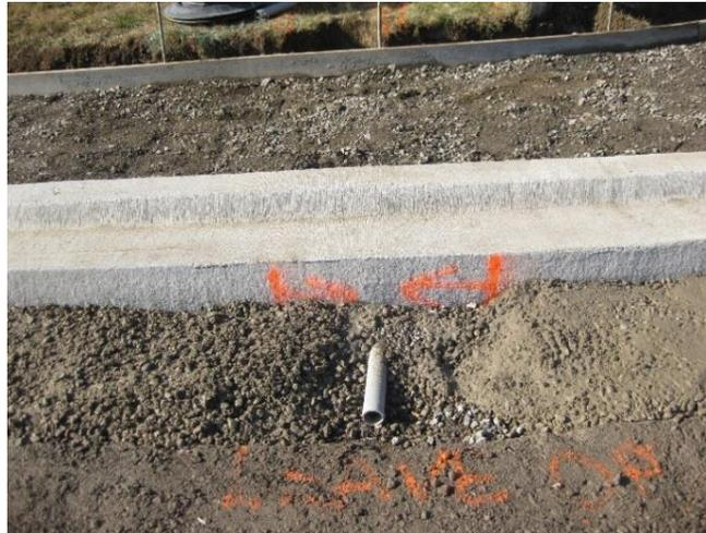
**Figure 4-12 PVC pipe below sidewalk for instrumentation**
