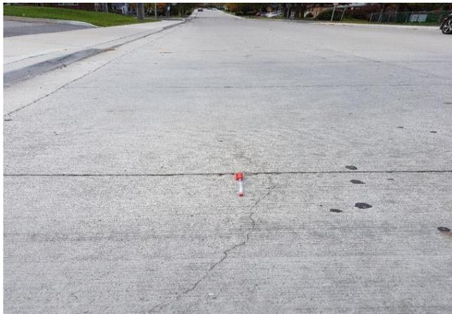
**Figure 5-32 Longitudinal cracking with slight meandering – Section 3 – 1Y after construction**
