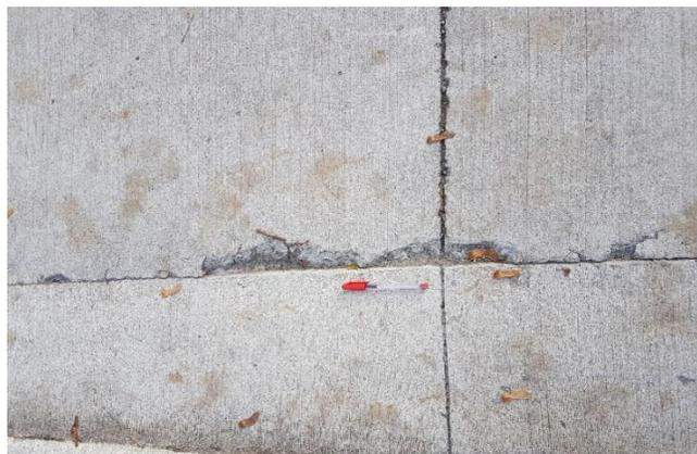
**Figure 5-28 Moderate longitudinal joint spalling – Section 2 – 1Y after construction**
