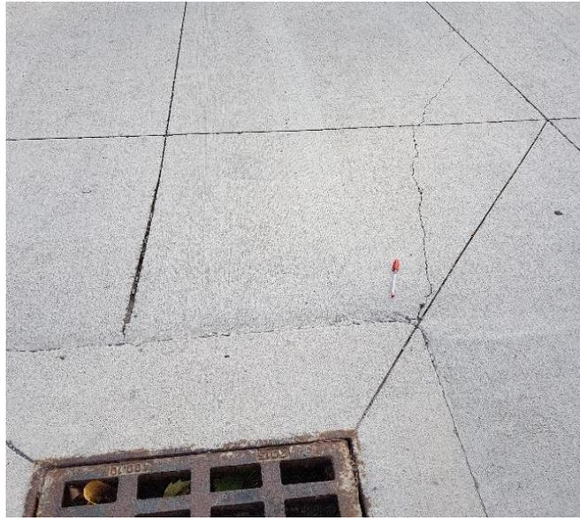
**Figure 5-27 Moderate transverse crack – Section 1**
