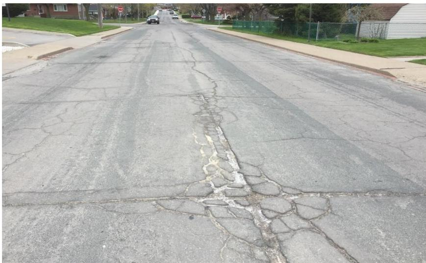
**Figure 3-6 Longitudinal cracks along Jameston Ave. (Pickel, et al., 2016)**
