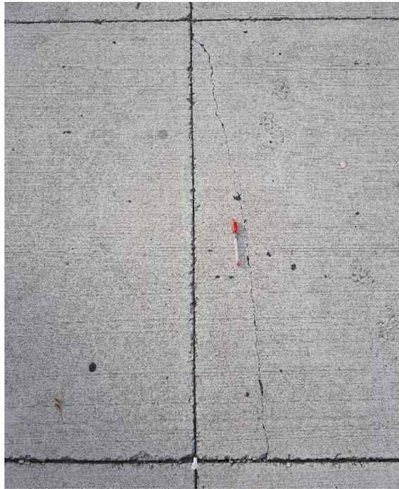
**Figure 5-30 Moderate longitudinal crack – Section 2 – 1Y after construction**
