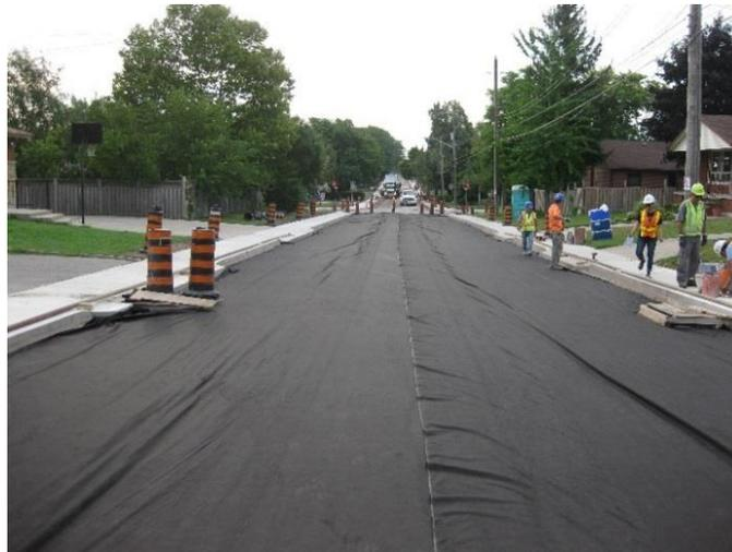
**Figure 4-13 Placement of geotextile on Section 1**
