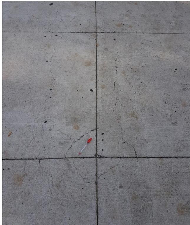
**Figure 5-29 Moderate d-cracking in Section 2 – 1Y after construction**
