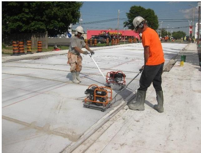
**Figure 4-20 Soff-cutting of longitudinal and transverse joints**
